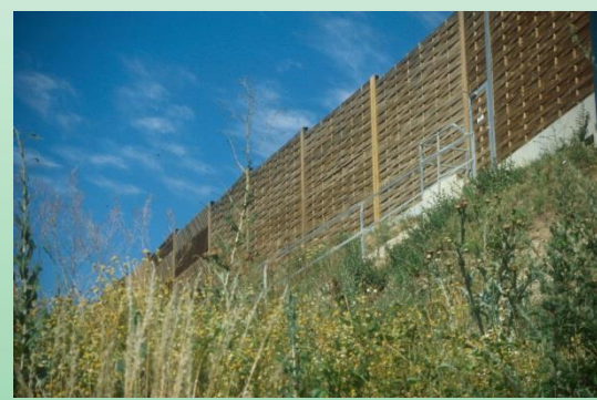
Noise protection wall in Lower Austria © Umweltbundesamt
