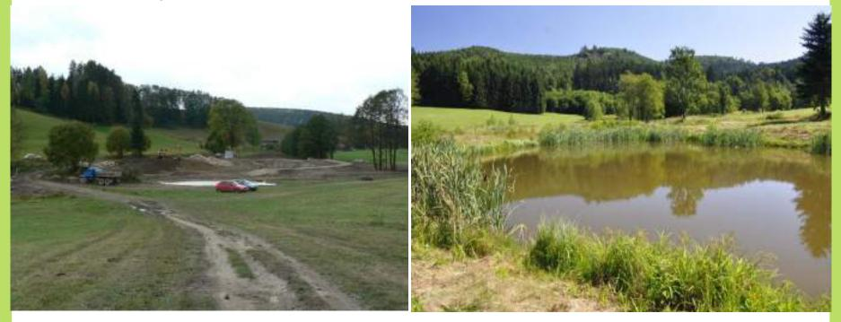
Construction of side water reservoir within revitalisation of water stream in Broumov region; similar small water reservoirs have no influence on the runoff balance, but are crucial for keeping microclimate and biodiversity in landscape; may serve as water sources for fire brigade
