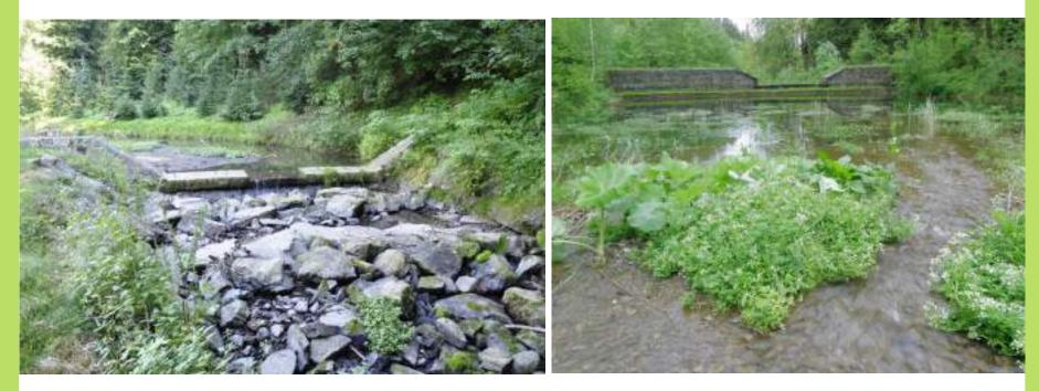
Retention constructions to held floating materials at Bohdašínský Stream and Kamenický stream (Rychnov Region); during minimum flow rate retention constructions might provide for survival of water organisms.
