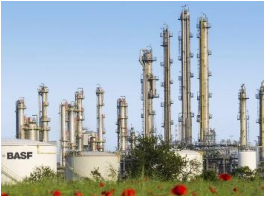
BASF: Oil as feed for Verbund
